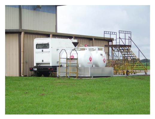
Photograph 6. Diesel and waste oil ASTs at heliport
